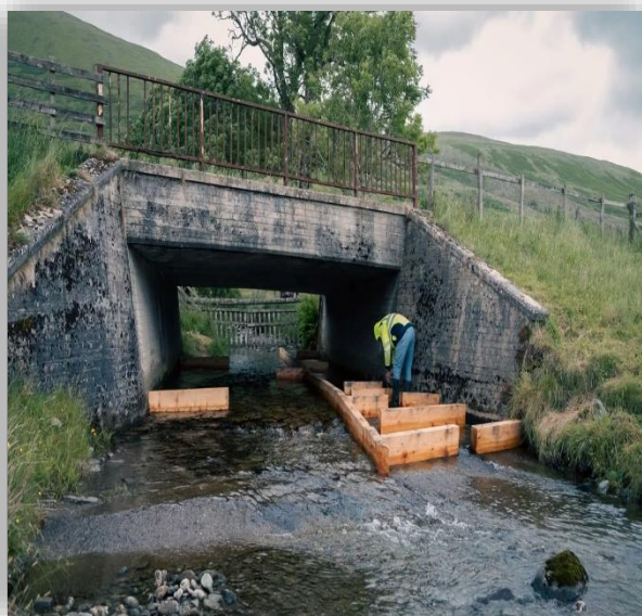
Fish passage installation on a bridge culvert in the Glen Fruin
